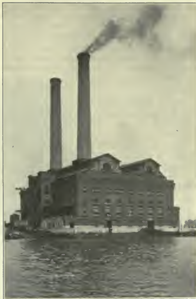
FIG. 487. POWER STATIONS. Steam Power Station, Port Morris, New York City, New York Central & Hudson River Railroad.
